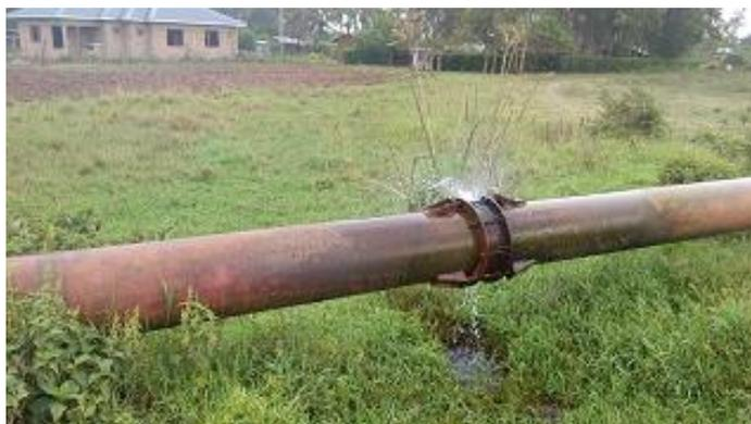
**Figure 2.9:** A burst section of the existing water pipe
