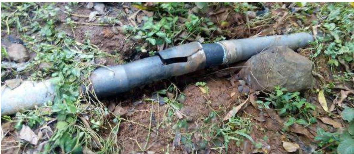
**Plate 4.2:** A dilapidated water pipeline from the Irate – Nginda scheme which is prone to damages, bursts and leaks in the rough terrain
