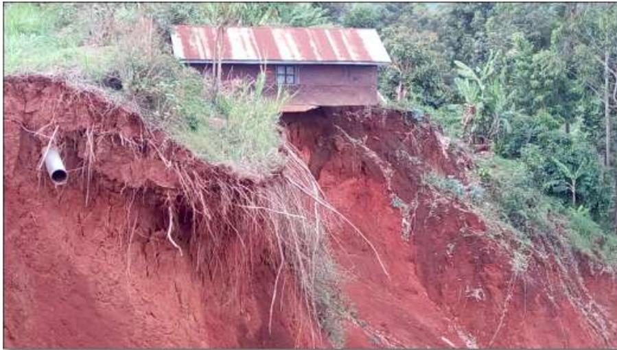
**Plate 4.1: Photograph shows a landslide that occurred away from the project site resulting in pipeline disconnection.**
