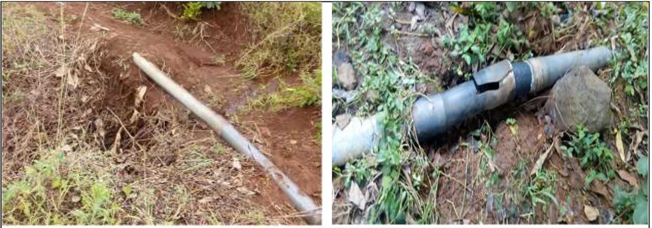
Plate 5.1: Dilapidated Irate Line Exposed Section
