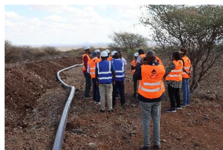
Inspection of pipe laying works under Kamboe Furmasan Water Project under HoAGW4RP
