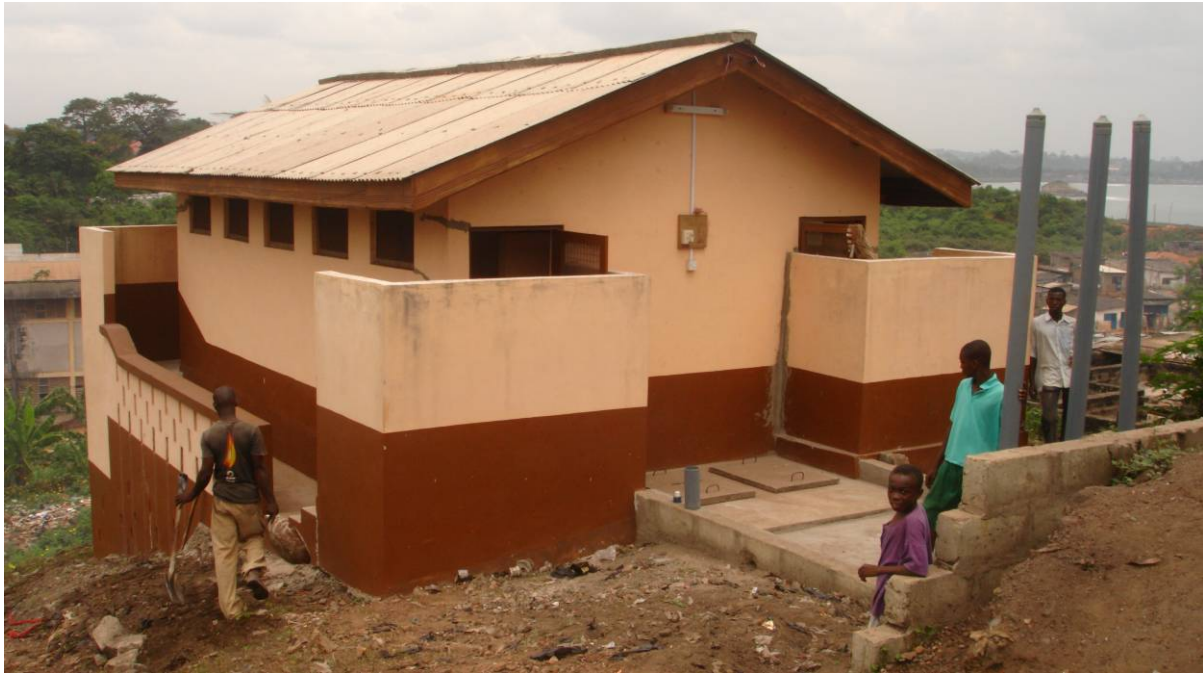
Figure 5: A JAFED Communal Toilet under Construction in Takoradi
